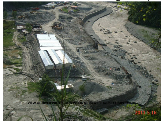
View of River Protection Work at Power House Complex
