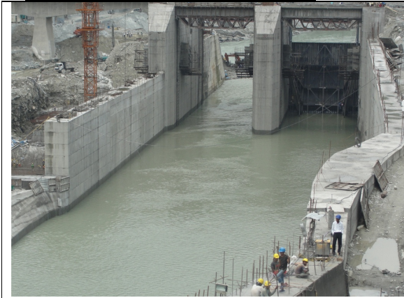
The Teesta River flowing through the barrage after phase 2 river diversion
