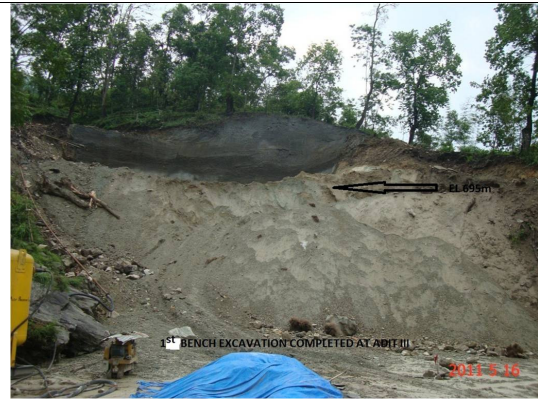
1 st Bench Excavation Completed at ADIT III
