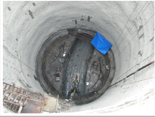
View from Surge Shaft top showing trench / HRT
