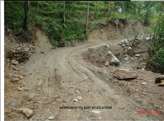
Approach to ADIT III Location
