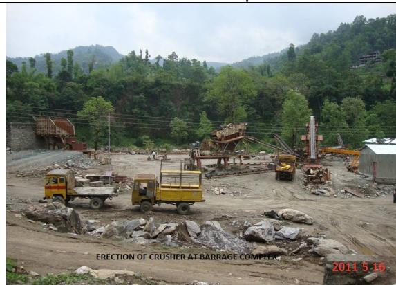
Erection of Crusher at Barrage Complex
