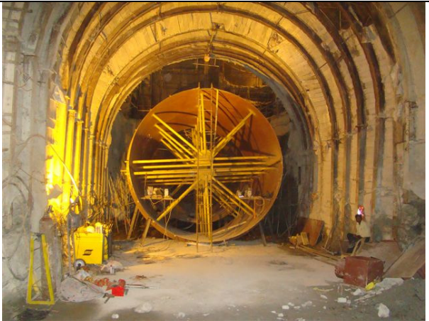
Erection of draft tube at unit 2 in the Power House Complex
